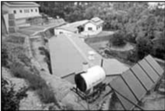
Solar water heating system
