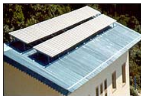
Photovoltaic solar panels for harnessing solar power
