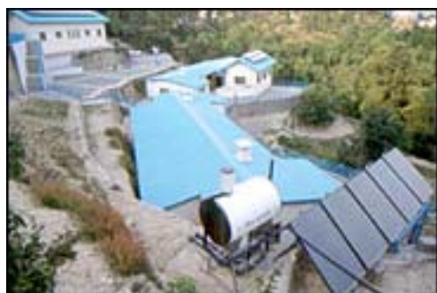
Solar water heating system
