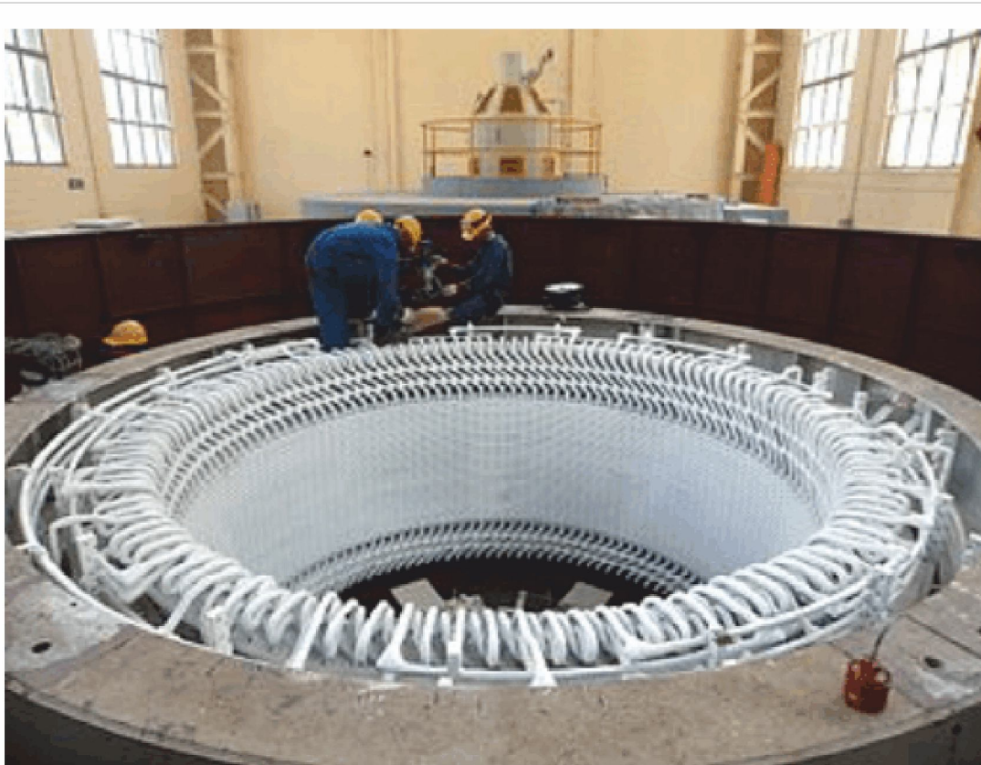
Figure 7: A large generator with the rotor removed
